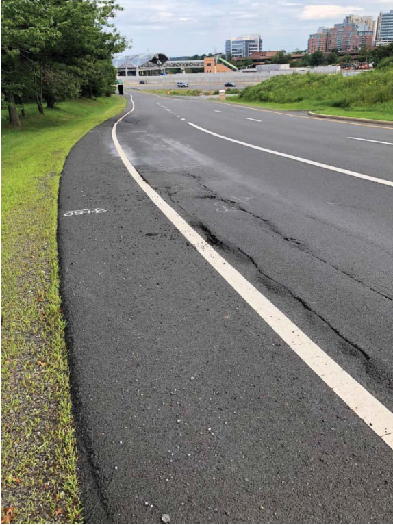
Photo 1: Example Cracking
